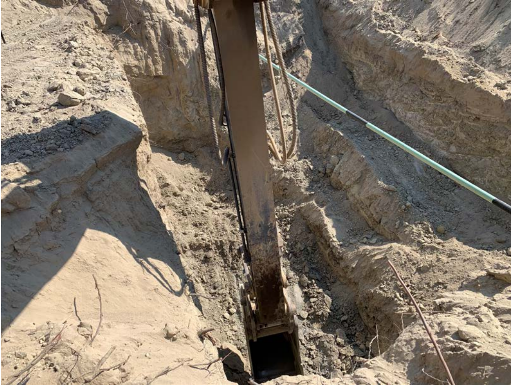
Photo 3: Final excavation extents, October 5, 2020.
