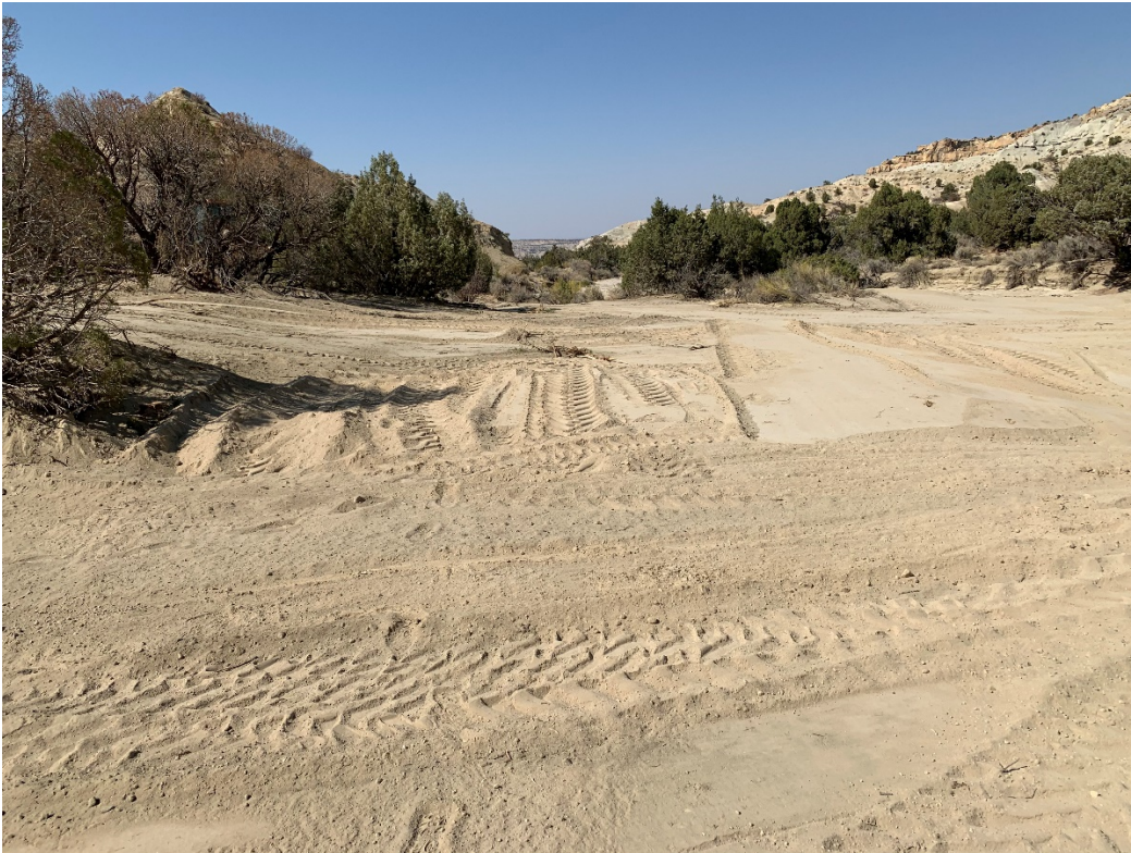
Photo 4: Backfilled excavation, October 7, 2020.
