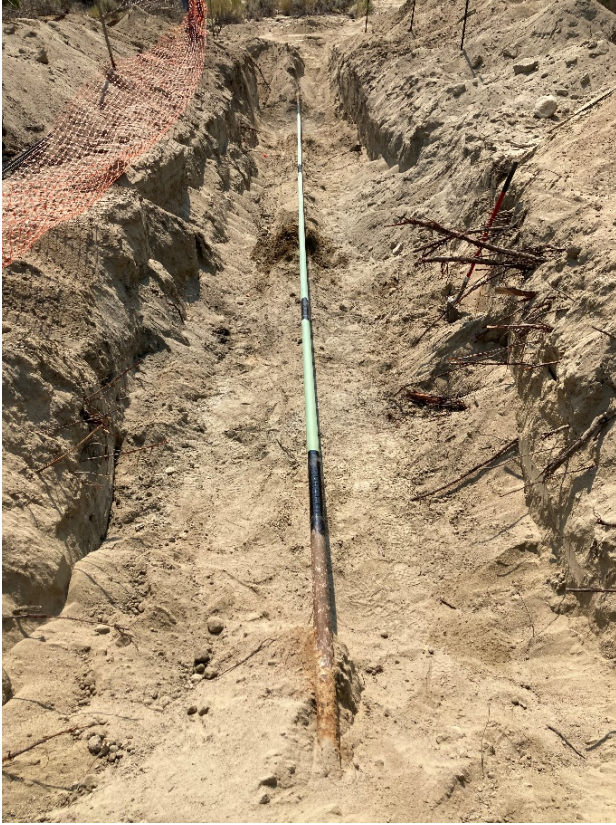
Photo 1: Excavated pipeline, October 1, 2020.
