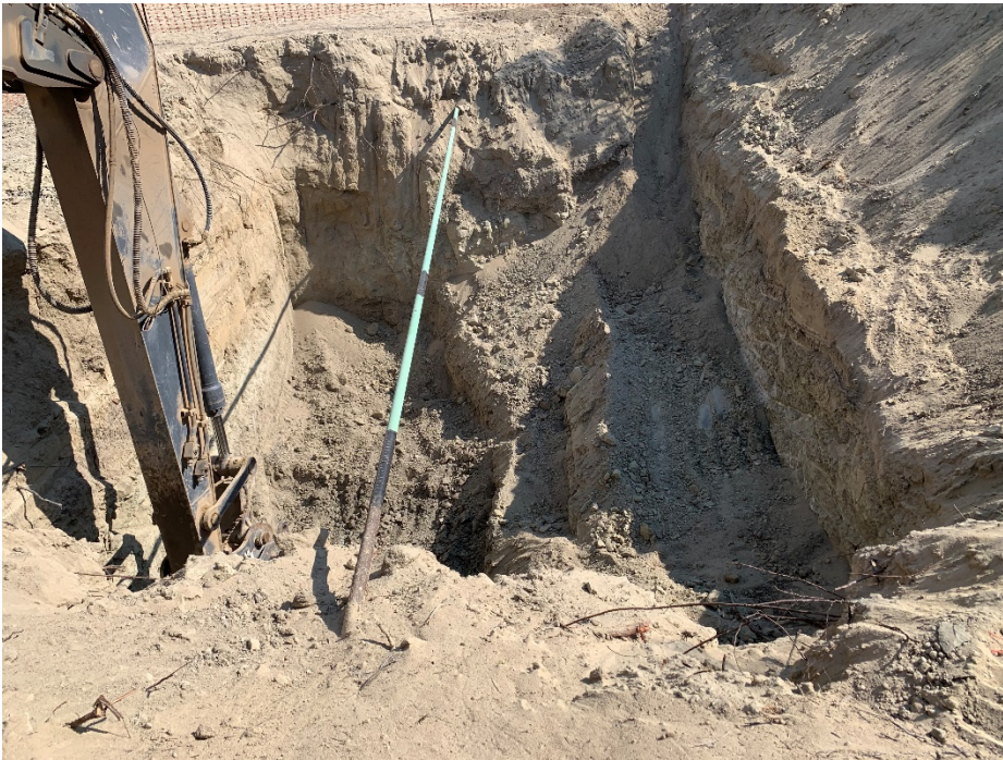
Photo 2: Final excavation extents, October 5, 2020.
